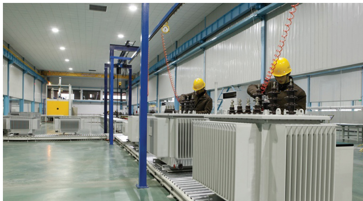
Amorphous oil-immersed transformer production line
