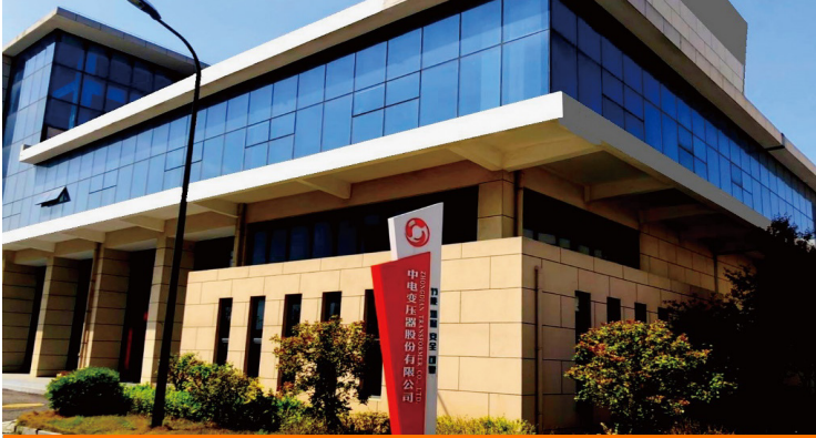
Zhenjiang Jurong Transformer Production Bases
