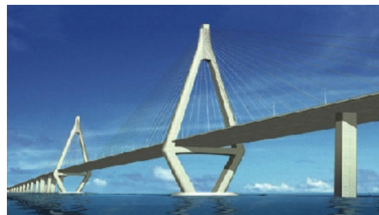
Hong Kong-Zhuhai-Macao Bridge
