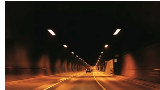
Shanghai Expo Huangpu River-Crossing Tunnel Project
