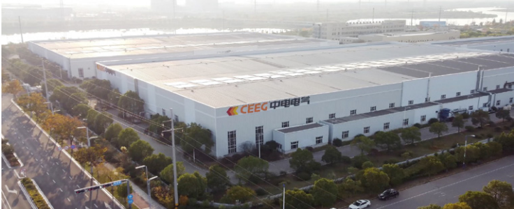
Nanjing Binjiang Production Bases
